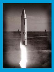
The Jupiter IRBM program enjoyed an impressive career in Cape history, from the earliest missile testing to Apollo 7. America's first successful full-size reentry vehicle in space launched on a Jupiter. The earliest bioflights, satellites, and space probes launched on Jupiter variants. Even Saturn I included a Jupiter tank core on its first stage, connecting the Apollo Program to Jupiter's impressive resume.
