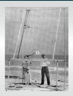
Prior to the use of our sophisticated tracking systems for rocket launch activity, sky screens were employed for range safety. They took many forms, but mainly consisted of two vertical parallel wires in a frame on a stand. The sky screen would be positioned a mile behind the launch pad with an operator calling out the track of the rocket/missile to a Range Safety Officer.
