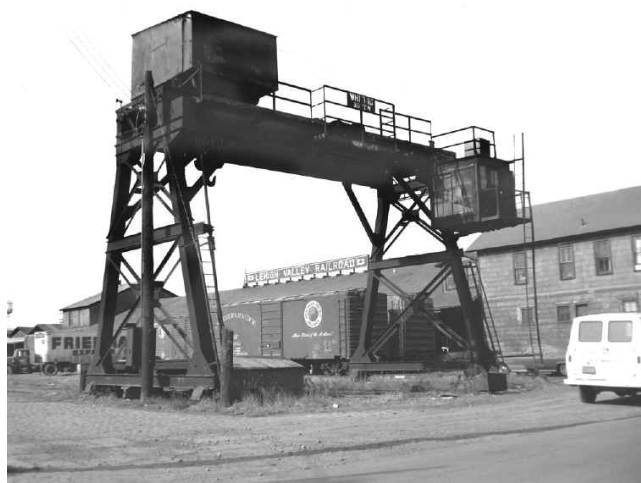
Gantry crane at the Wilkes-Barre CNJ rail yard
