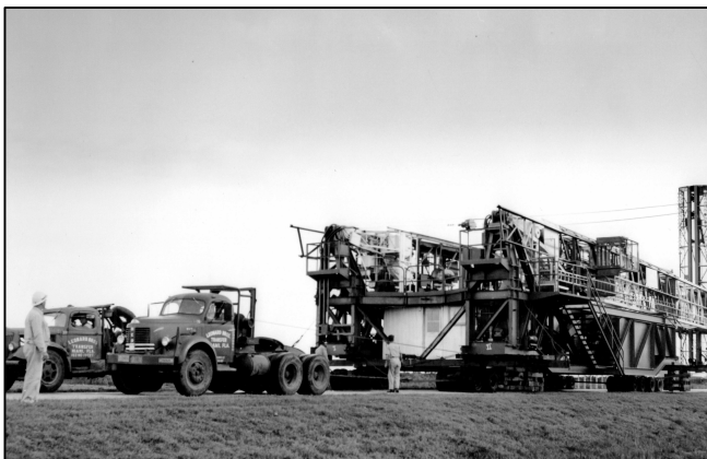
Launch Complex 4 gantry with mast lowered and ready to be towed to Launch Complex 5/6
