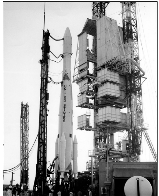
Delta 54 (E-1) on 10 November 1967 being serviced by the modified gantry on SLC-2E.
