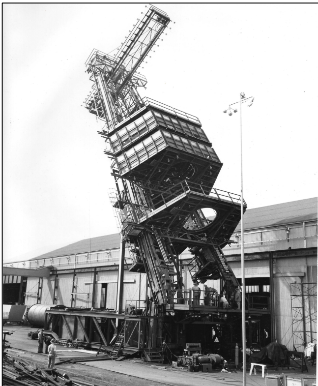
The gantry self-erecting mechanism being tested at the Noble facility (Credit: Pete Noble)
