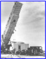
MINUTEMAN TRANSPORTER/ERECTOR ALIGNED WITH SILO 31
