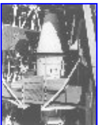
MIDAS NOSE SECTION IN PLACE ON GANTRY AT PAD 14
